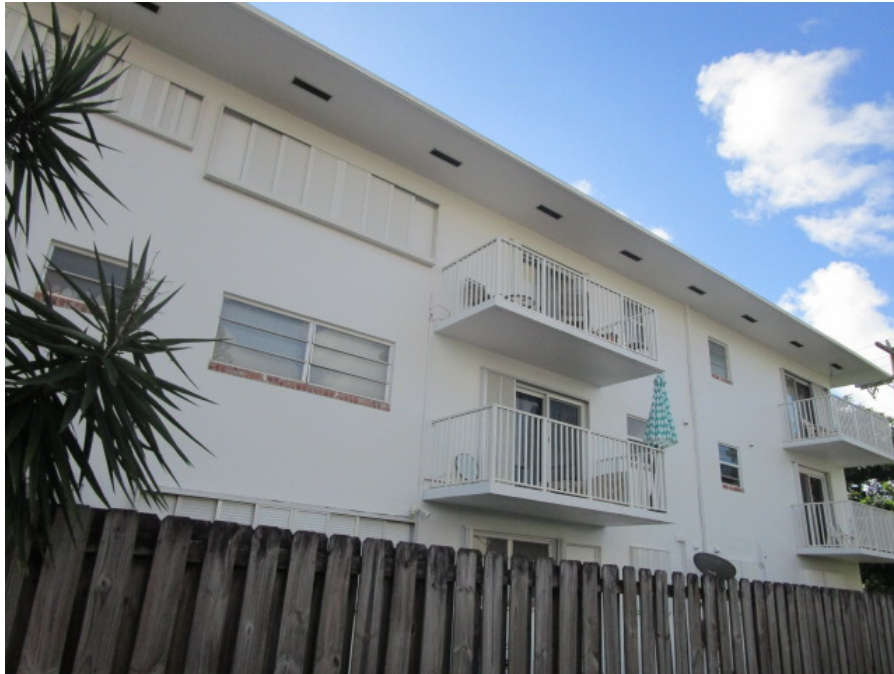
Photograph #003 Overview of main building
