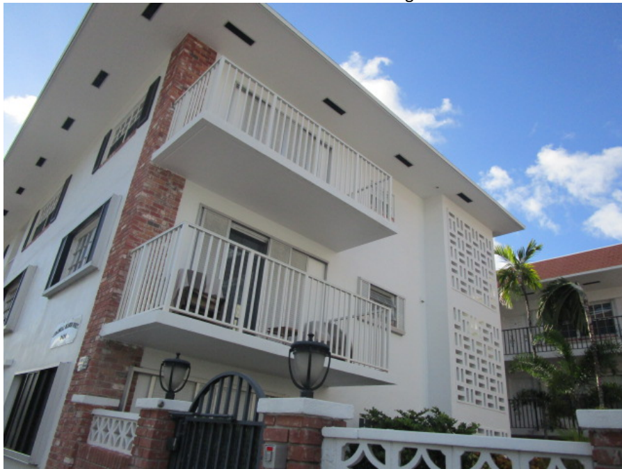
Photograph #004 Overview of main building
