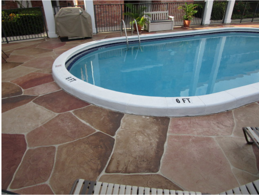
Photograph #005 Overview of pool/ pool deck.
