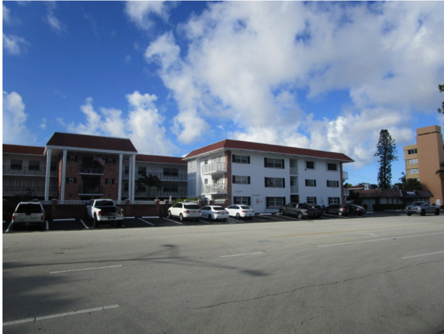
Photograph #001 Overview of main building
