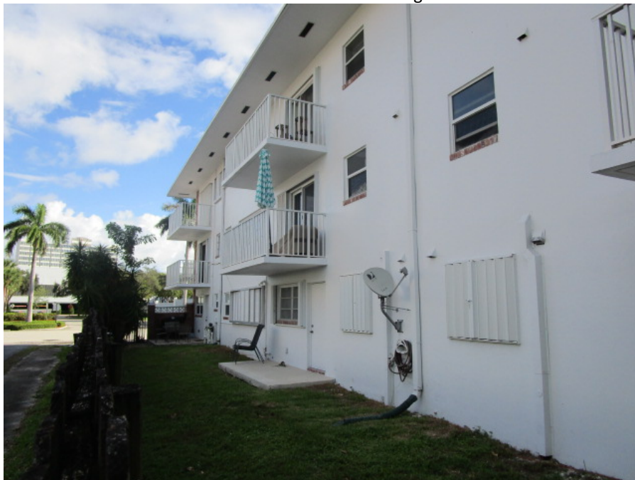
Photograph #002 Overview of main building
